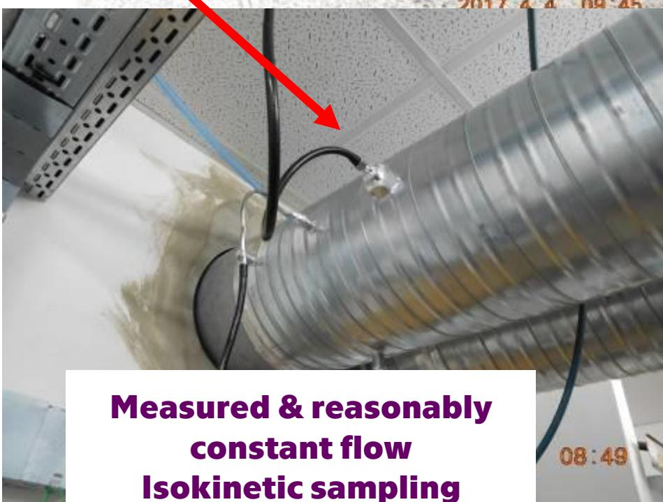
Measured & reasonably constant flow Isokinetic sampling
